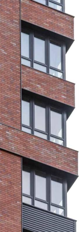
Brick to Click combines the outstanding properties of clinker with the typical advantages of a ventilated curtain facade in a facade cladding.
